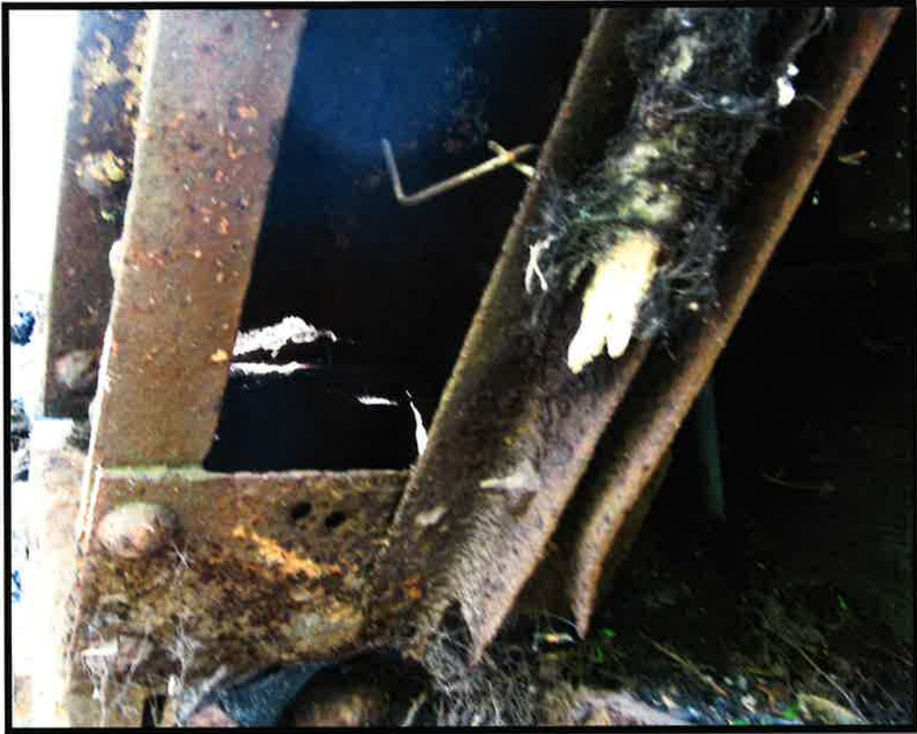
Southwest bridge seat under view (note poison ivy root system) Northwest Corner
