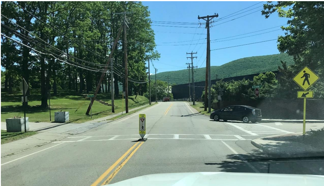
In-Street-Yield Sign (MUTCD R1-6) in the crosswalk on Rt. 52 at Blackburn Avenue/Robert Cahill Dr. Installed on May 27, 2021.
