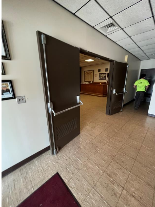
Dark Brown Cove Base Molding Positive for Lead
