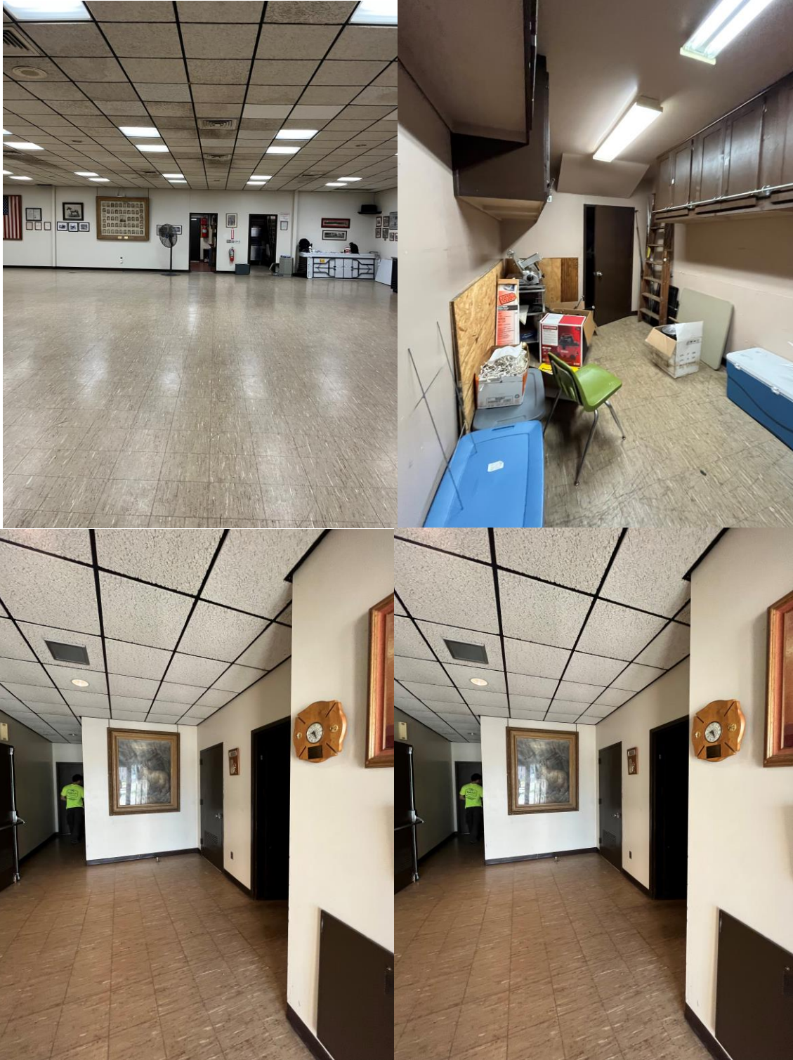
ACM Floor Tile Throughout Lower Level
