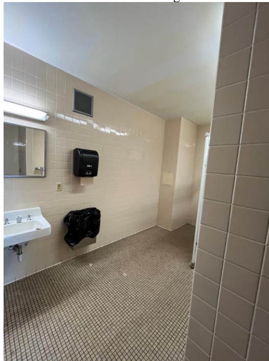
Ceramic Wall Tile & Sinks Positive for Lead in All Bathrooms
