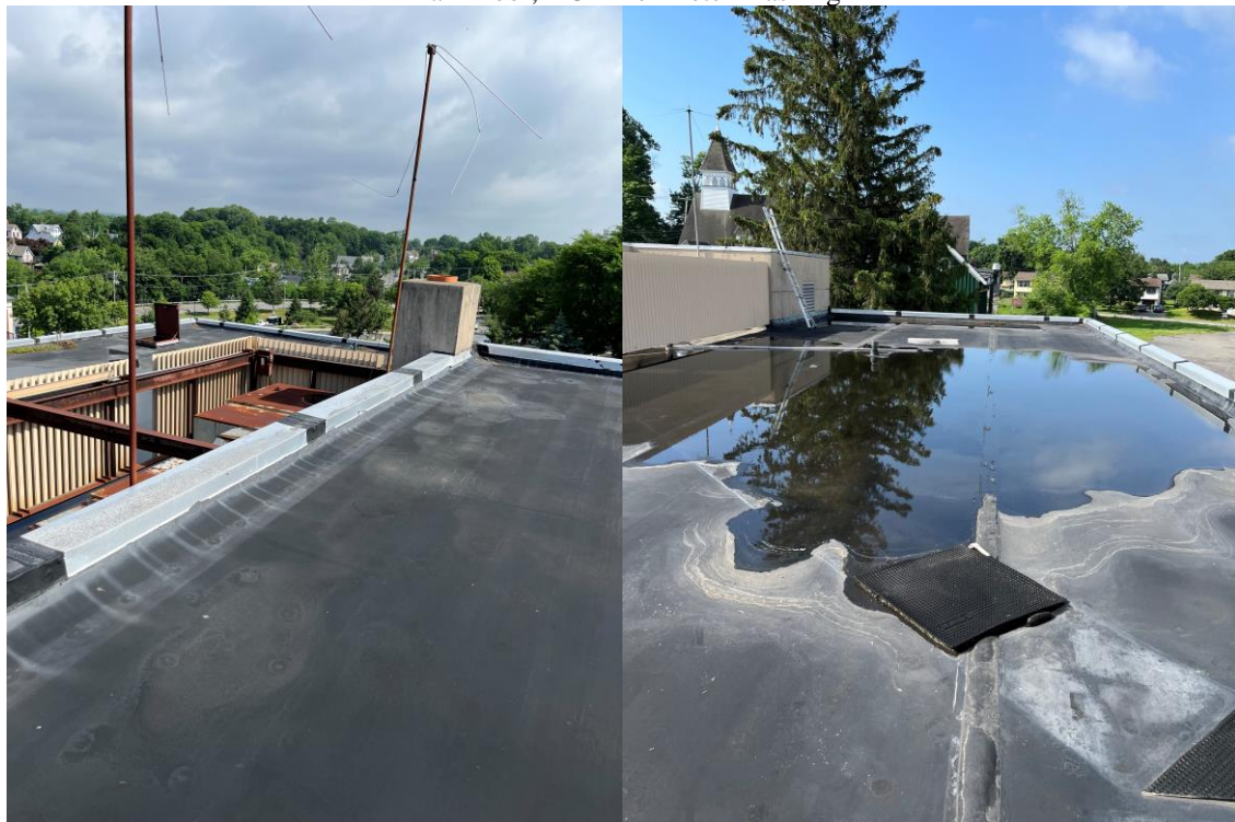
ACM Termination Caulk & Tar Under Coping Throughout
