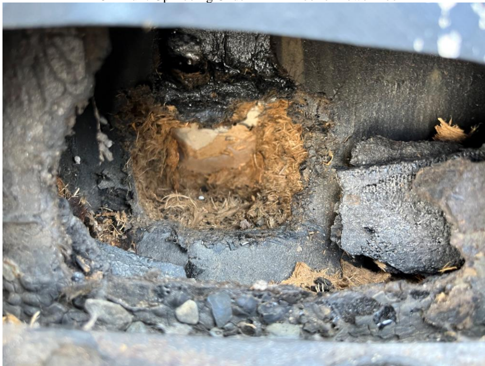
ACM Building Flashing on Lower Roof
