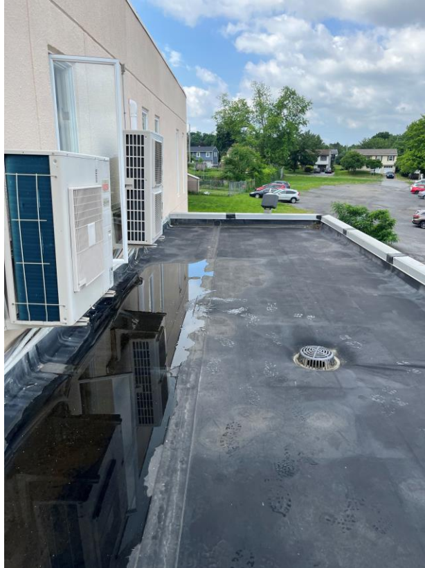
ACM Built-Up Roofing Under EPDM Roof of Lower Roof
