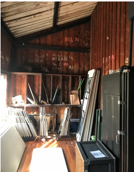
Front utility room
