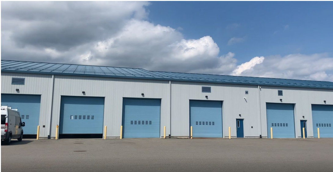
Southeast-facing roof at 30 Camp Beacon Road
